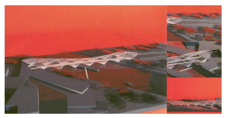
The structural functioning of the chosen solution is that of a reticulated multi-span vault. It is well known that the behaviour of vaults is highly adequate to solve the problem of great spans versus distributed loads.
